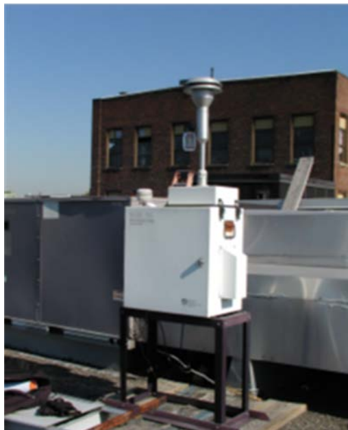
Figure 2 Photo of USEPA-approved PM 2.5 sampler on the roof of the Union City Health Department building in Hudson County
